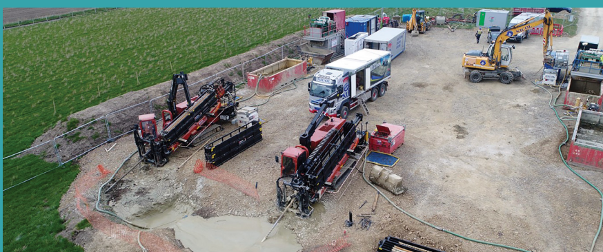
Illustrative image of Horizontal Directional Drilling on temporary construction compound.
