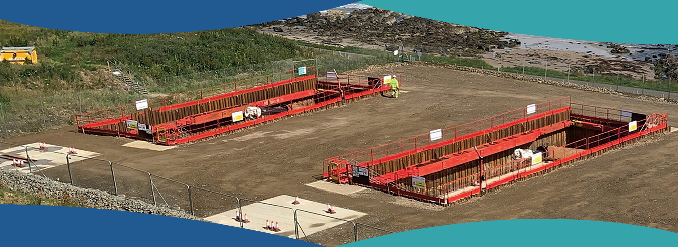
Typical landfall compound with two Transition Joint Bays ready for cable pull-in.
